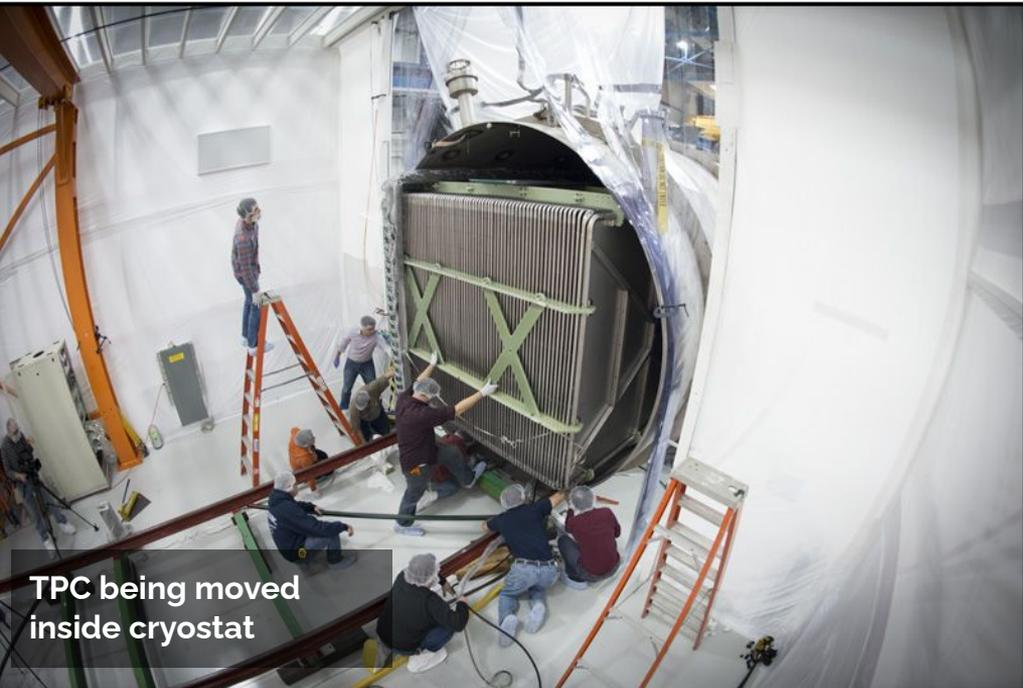
TPC being moved inside cryostat
